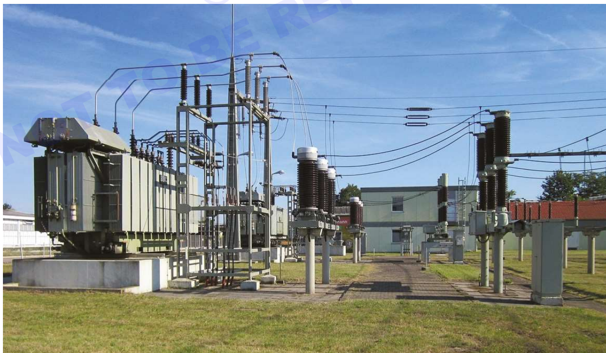
DISTRIBUTION SUBSTATION
