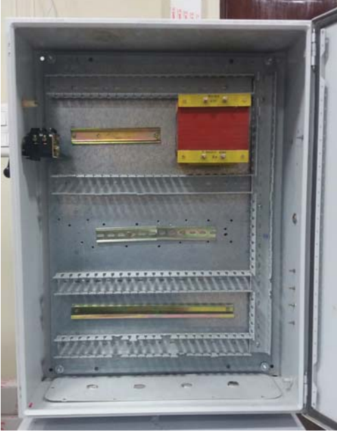
CONTROL PANEL WITH RACEWAYS/DIN RAILS
