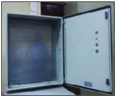
CONTROL PANEL WITH MOUNTING AND FIXING HOLES
