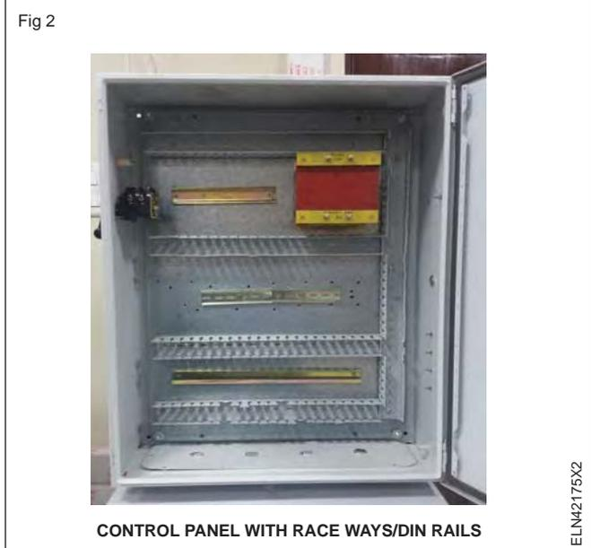
10 Fix the race ways, DIN rails and G channel using fixing screw.
