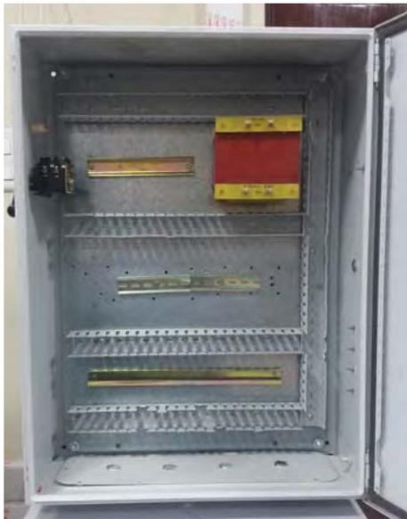
CONTROL PANEL WITH RACEWAYS/DIN RAILS
