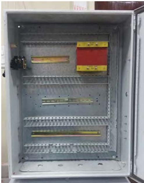
CONTROL PANEL WITH RACEWAYS/DIN RAILS
