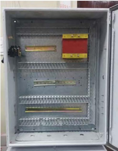
CONTROL PANEL WITH RAYS/DIN RAILS
