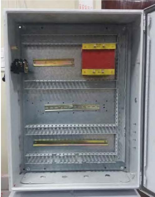
CONTROL PANEL WITH RACEWAYS/DIN RAILS
