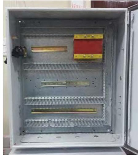
CONTROL PANEL WITH RACEWAYS/DIN RAILS
